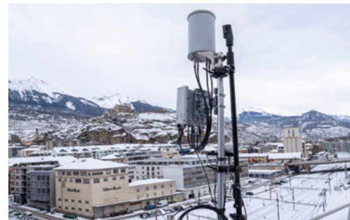
The mobile antenna with 5G micro remote radio head
