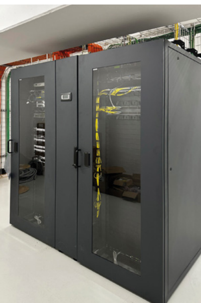
The SMDC in Montecavolo, the Granterre site in Reggio Emilia
