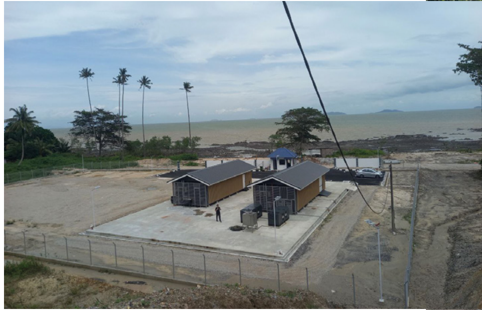
The cable landing station at the Mersing site
