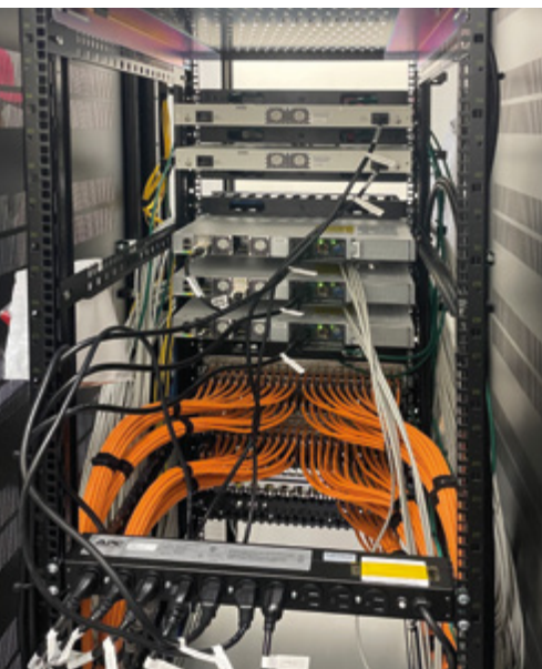
Network rack with copper and fibre optic connections
