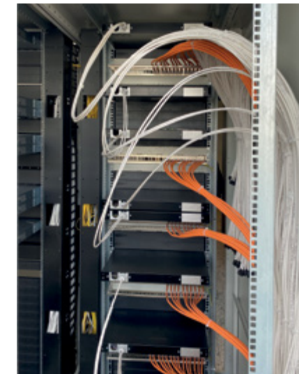
Copper and fibre optic panels in a data distribution room
