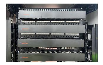
The structured premises cabling comprises 13,800 Category 6 copper data connection points, and the installation involved exclusively cables with LSZH sheaths. Not only is the entire communication technology integrated
