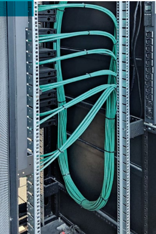
Installation of fibre optic cables in the rack
