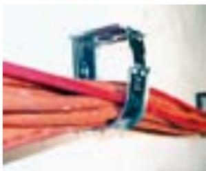
After installing the cable, close the Hermann clip using the integrated folding mechanism.
