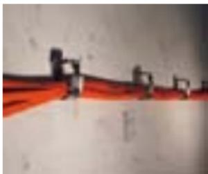
The universal "Hermann clip" can be installed on walls or ceilings. The cover is always situated on the side and the rounded cable support surface always faces downwards.
