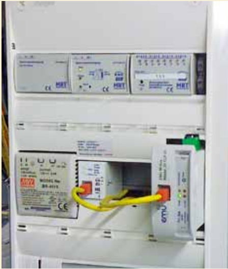
带有VaserControl MiniBox的系统装置在BZT里的表面固定盒中 System devices with VaserControl MiniBox in surface-mounted box in the BZT.
