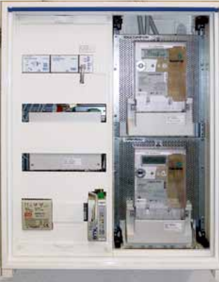
带有系统装置和KNX三相变压器表的表面固定框架 Surface-mounted frame with system devices and KNX electrical 3-phase transformer meter.
