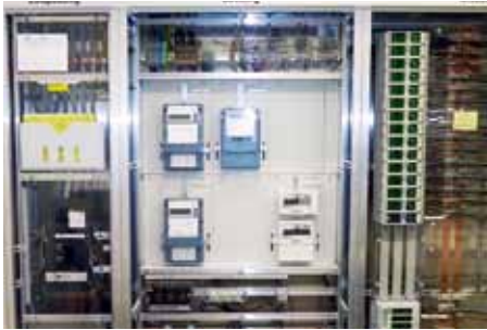
在州档案馆中的主配电板 Main electric distribution board with transducer in the State Archive.
