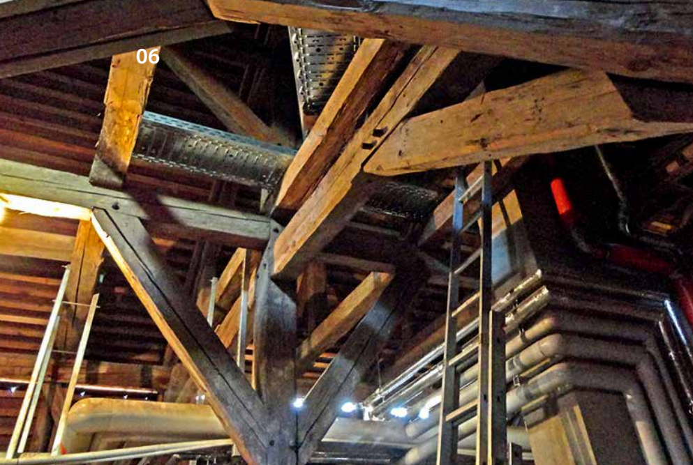
在修道院阁楼内，将光纤环网沿着线缆托架设置 The fibre optic ring is routed along cable trays in the attic of the convent buildings.
