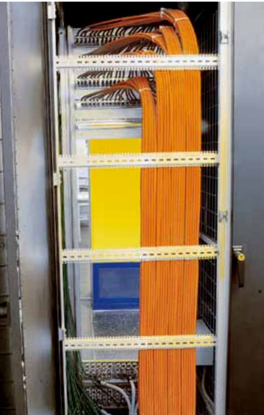
从里面看分配器机架：最佳的电缆路线安排。 Distributor rack from the rear: optimum cable routing.
