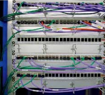
安装进现有机架内的新布线。 The new cabling fitted into the existing racks.
