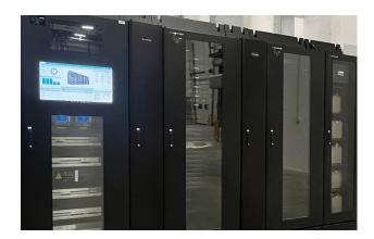
This included the integration of various systems such as power distribution, air conditioning, UPS and batteries as well as monitoring and Cat.6<sub>A</sub> cabling.
